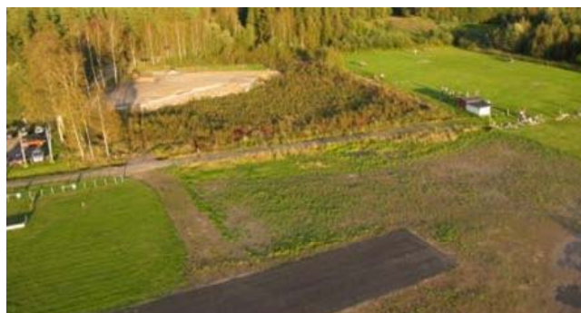
At the top you can see the almost finished tarmac circle for F2A and F2C. To the left you find all buildings and the grass circles can be seen in the upper right corner.
